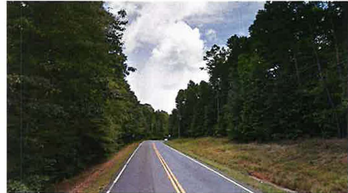
EXISTING HIGHWAY 53 NORTH
