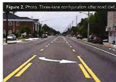
Figure 2. Photo. Three-lane configuration after road diet. Source: Pedestrian Bike Information Center, "Road Diets" training module, 2009.
