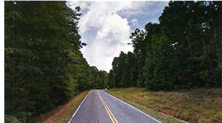
EXISTING HIGHWAY 53 NORTH
